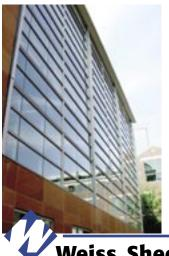
Accent trims at the floor levels (top right) and sun shades which extend from the buildings facade create a unique look the architect desired for Harvard's, Naito Chemistry building (above and right). Weiss was also tasked with the creation of custom fabricated stainless steel brackets to securely hold the sun screen fins in place. Custom Verticals were also used (left) which angled out slightly from the curtainwall facade.
