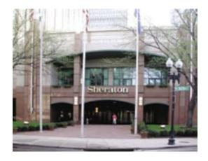
A custom matched, forest green paint was required for the radiused aluminum panel accents on the 2000 Sheraton Hotel. Large archways enhanced the entrance while smaller spans were required for the windows. Lighting units were incorporated into the final design of the archways which kept the recessed window units bright and highlighted the red stone of the facade.
