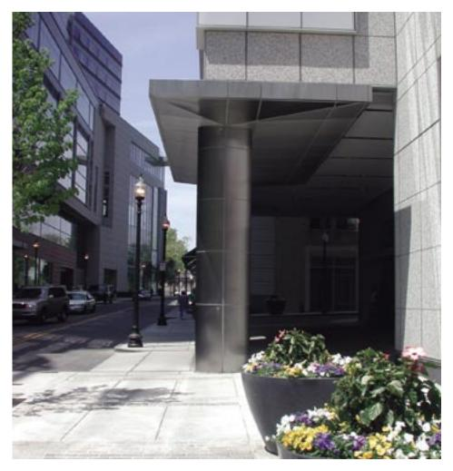
Making perfect mitred joints then welding and polishing, Weiss achieved the desired results. For this project, Weiss worked with a # 4 satin finished stainless, but they also have the ability to work with #6 and #8 "mirror" stainless.
